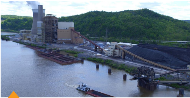
Cardinal Power Plant | Coal-fired power plant Brilliant, Ohio | 1,230 MW capacity
