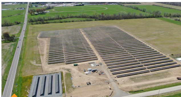
OurSolar Up to 4.76 MW of solar energy output from 24 arrays across Ohio. The newest, and largest array, OurSolar2, went live in July 2022, with nearly 8,000 new panels, generating 2.66 MW of solar power generation.
