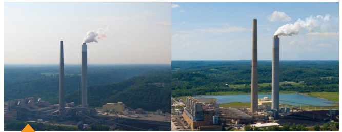
Ohio Valley Electric Corporation Clifty Creek Station, Madison, Indiana Kyger Creek Station, Cheshire, Ohio Coal-fired power plants | 434 MW combined capacity
