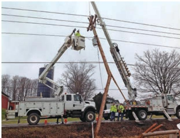
HWEC linemen work diligently to replace a broken pole from a car accident on State Route 83.
