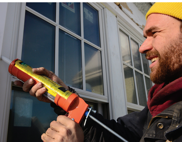
The average American family spends $2,000 annually on energy bills, but unfortunately, much of that money is wasted through air leaks in the home. Applying caulk around windows, doors, electrical wiring, and plumbing can save energy and money.
