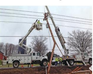
HWEC linemen work dilegently to replace a broken pole from a car accident on State Route 83.
